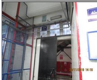
Photo of non-conformity Emergency exit slide door type - washing section.JPG
