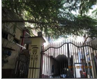
External photo(s) of the production unit(s) Facility building outer view.JPG
