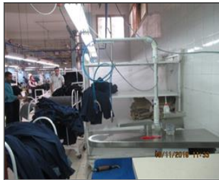
Photo of non-conformity Stain removing open to production section and not isolated.JPG
