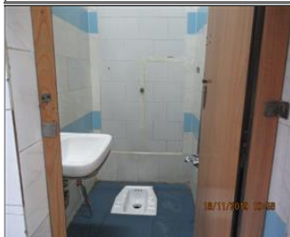
Photo of the sanitary facilities Toilet.JPG
